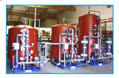
individual air solenoids for pneumatic valve actuation, system also includes continuous digital readout of step in progress and time remaining, panel-mounted conductivity monitor/controller with provision for pushbutton automatic or fully automation operation. Also incorporates battery back-up system to prevent loss of program memory due to power failure. Controller is housed in a NEMA-12 CABINET.
